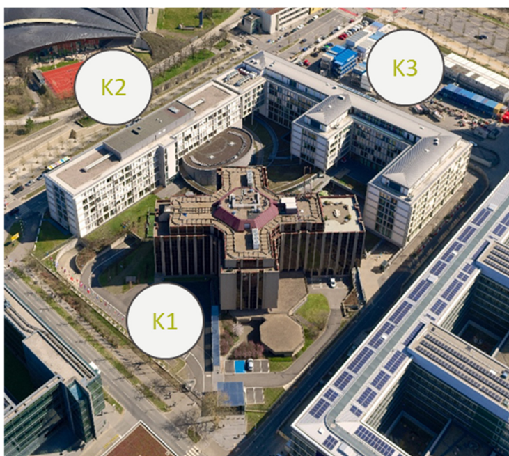
Figure 4 – Aerial view of the ECA’s buildings
