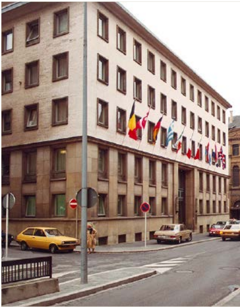
First ECA building, 29 rue Aldringen, Luxembourg
